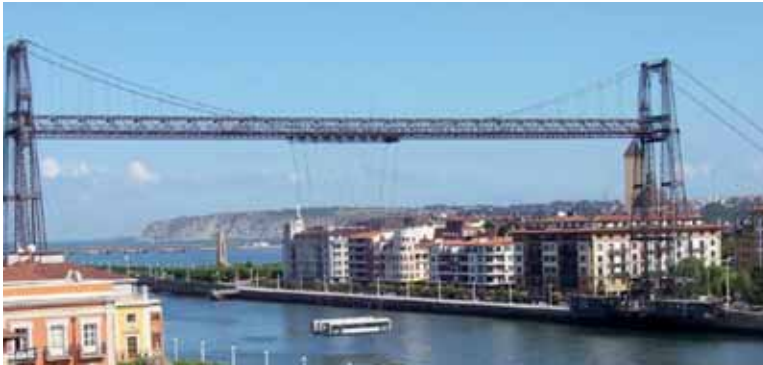
Portugalete's Vizcaya Bridge – the famous hanging transporter bridge (Puente Colgante) near Bilbao in the Basque Country
